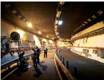
Works on the Sai Van Bridge tunnel
